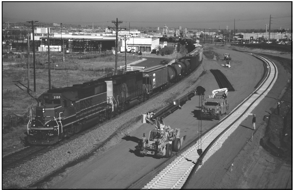
BNSF's Denver, CO, to Amarillo, TX, train with BNSF GP38-2 #3188 rolls south past new track alignment. The joint line is being relocated by RTD's Southwest Light Rail corridor. The Light Rail will be extended from South Broadway to Littleton. Workers were placing welded rail onto concrete ties at South Denver on 2/23/98 – Photo by Chip Sherman
